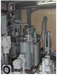
Before Retrofit - Hitachi Mechanical Cabinet Actuator
