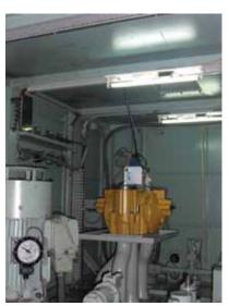
After retrofit - L&S Manifold & Distributing Valve mounted in the existing governor cabinet
